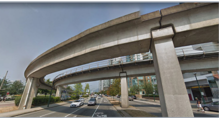
Curve guideway segment next to Science World Station
